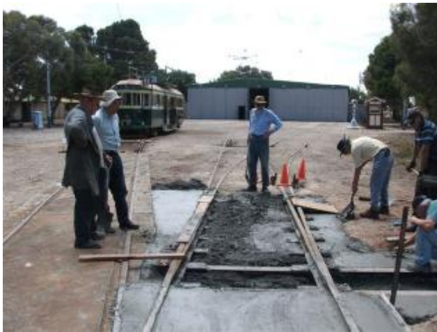
The laying of the concrete is progressing. Chris Summers
