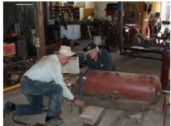
Bruce Lock and Michael Crabb making steel bands to support the air compressor tank for car 118 on Friday 16 Nov 07.
