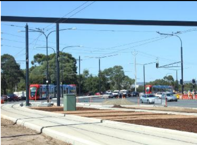
The Citidas on the left has just left the West Terrace stop for Entertainment Centre / Hindmarsh on the first regular service day, 22 March 2010. Another Citidas on the right is on the return journey. The tracks are widely spaced at this point to allow for the West Terrace shuttle terminal track in between them behind the photographer. Steve McNicol
