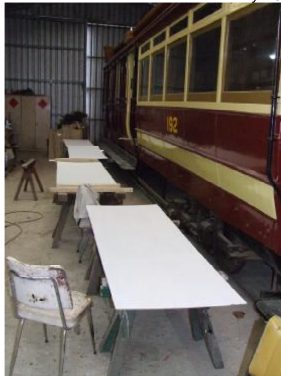
The ceiling panels being prepared for the saloon of No. 14. 192 currently stored in the Bodyshop to allow the Bib & Bub set to be located over the pit in Road 2.
