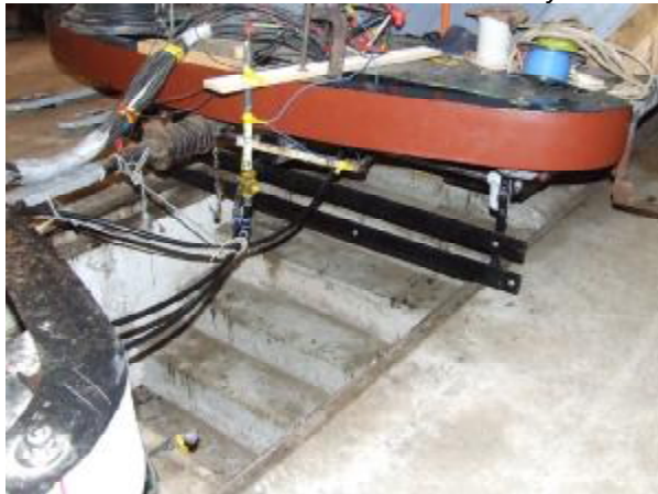
The equipment set up to test and validate the emergency stop system on the inner end of No. 14.
