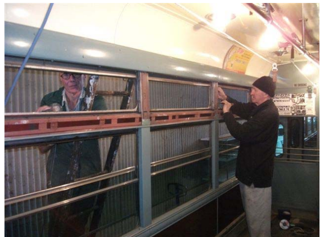
Charlie Rodgers and Bruce Lock working on 381 on 27 May 2011.
