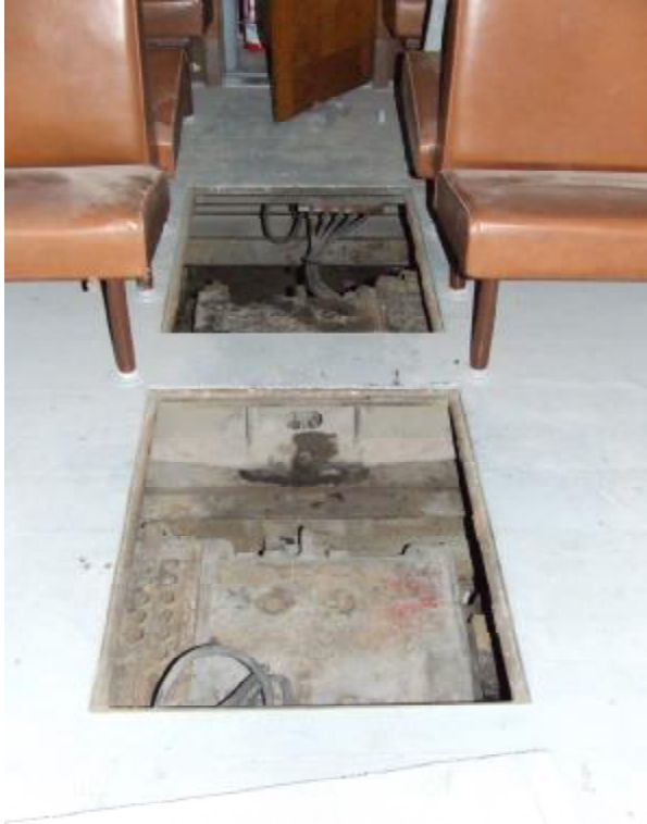
The new trucks as seen through the floor hatches on 1013.
