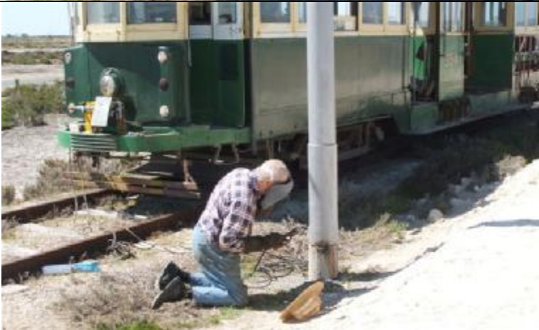
Bruce Lock welding the pole. Works car W2 354 provides the power.
