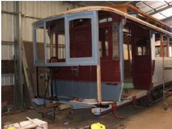
This photo was taken on 25/01/08. It shows car 14 a few days before installation of its K35JJ controller.
