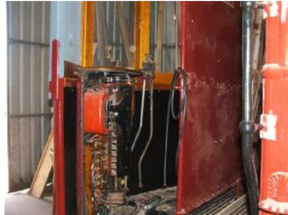
This photo was taken on 25/01/08 and shows car 118 with the GE B23 controller obtained from Victoria and installed 3 years ago, along with a brake valve installed in February 2008.
